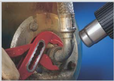
LOOSENING BOLTS AND RUSTED PARTS
